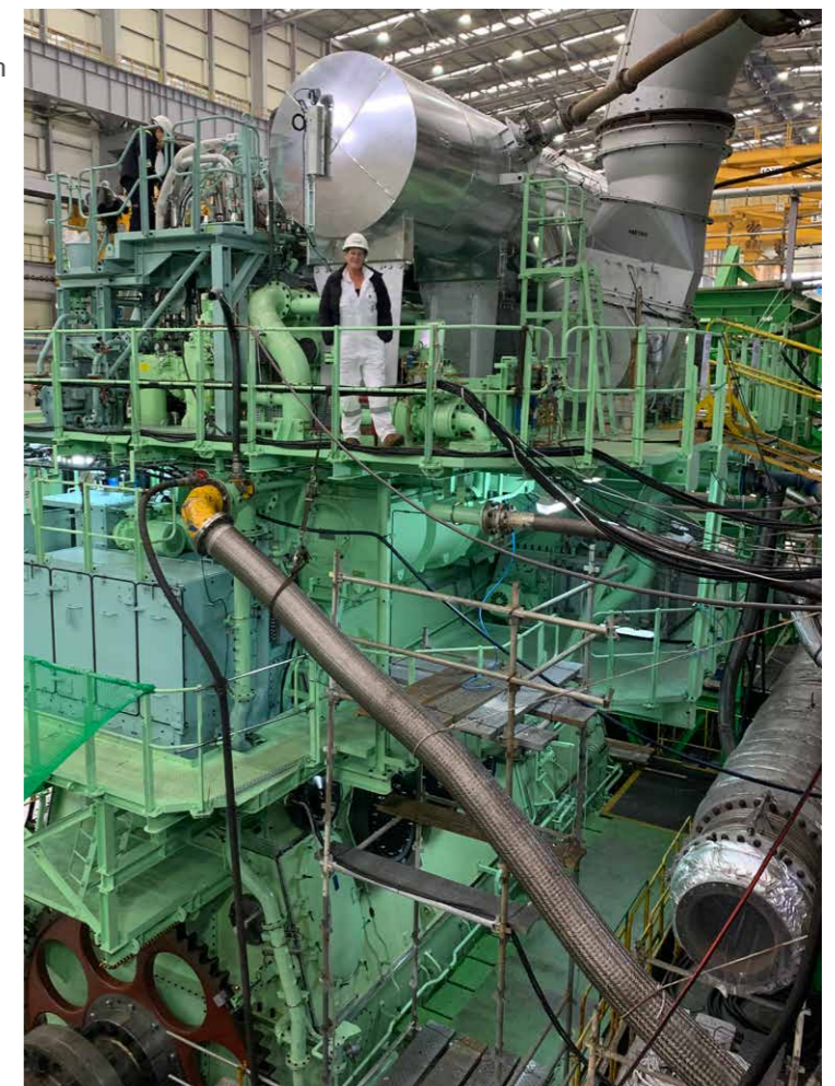
BW LPG Fleet Supervision Manager inspecting the LPG dual-fuel parent engine during final testing
